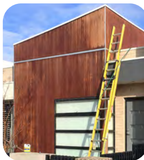
CLEANING: Wash the boards with a deck cleaner and a soft brush.
