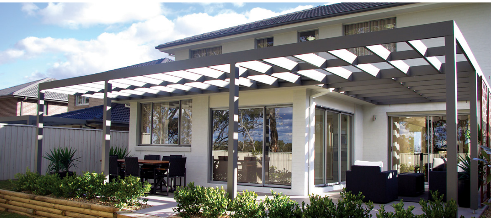
Posts, beams and rafters
