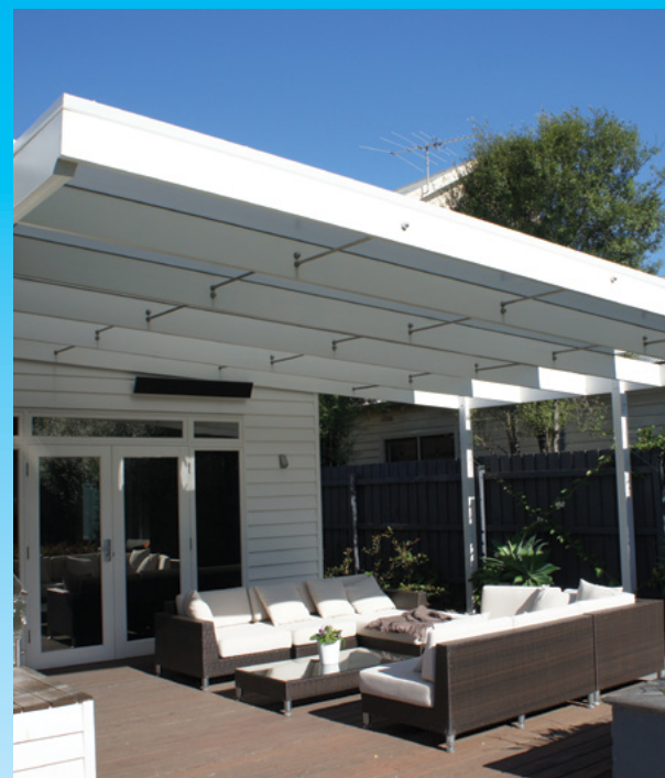
Posts and beams
